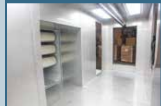
CLEAN INTERIOR FINISH
