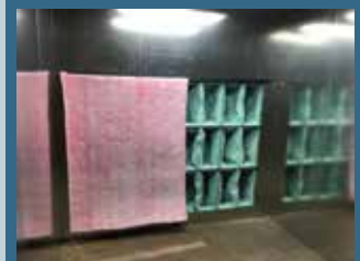
PRIMARY FILTRATION: BLANKET OVER POCKET FILTERS
